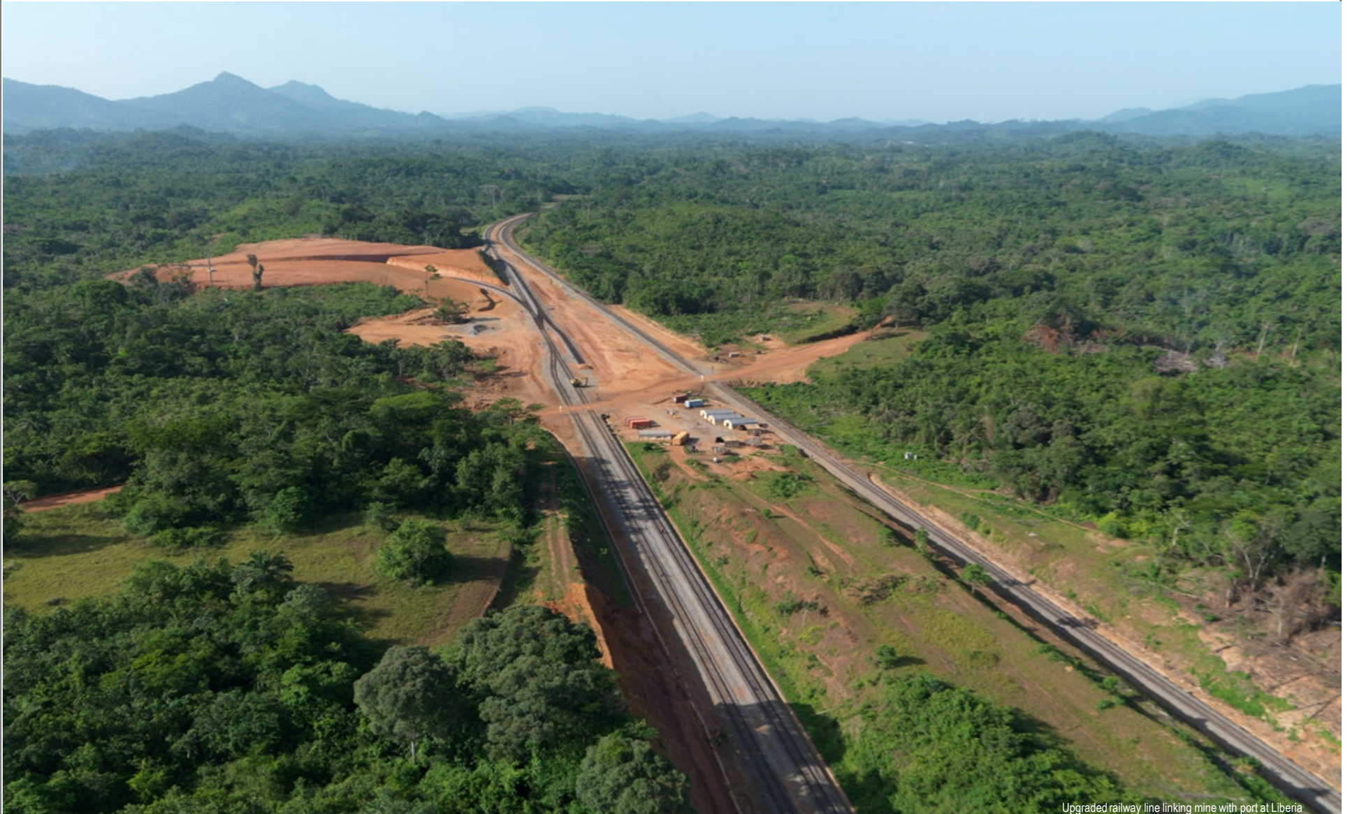
Upgraded railway line linking mine with port at Liberia
