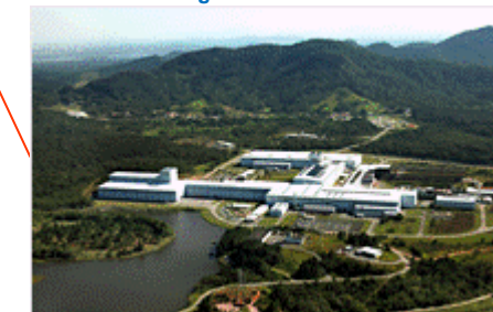
Finishing facility currently under expansion; post expansion, 1Mt of capacity
