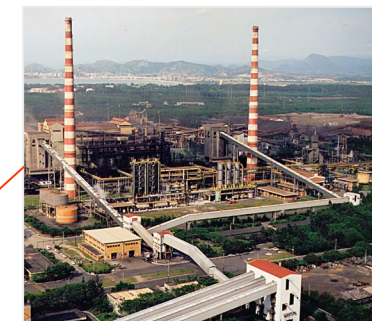
3BFs and 3 BOFs; 7.5Mt of annual slab capacity; HSM with 4.3Mt capacity
