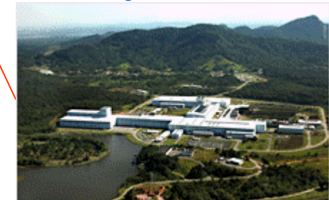
Finishing facility currently under expansion; post expansion, 1Mt of capacity
