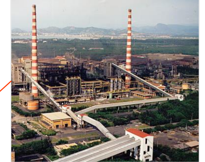
3BFs and 3 BOFs; 7.5Mt of annual slab capacity; HSM with 4.3Mt capacity
