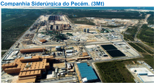
1 BF and 2 BOFs with 3Mt annual slab capacity
