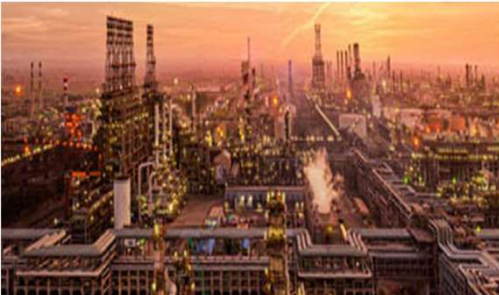
Reliance Jamnagar refinery expansion phase 2 (Oil Refinery) S420M - 10,811MT
