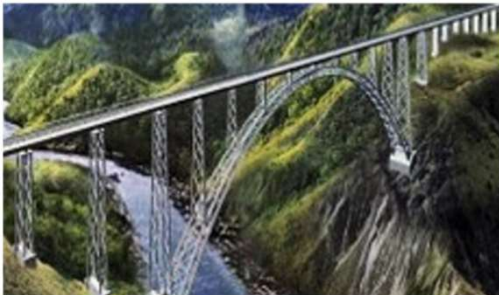
Chenab Bridge E410/350/250 - 25,000MT
