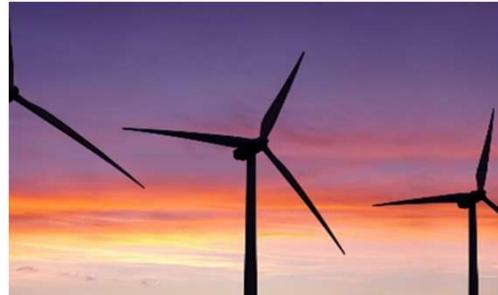
High strength structure (Wind Mill) S460ML - 3,600MT
